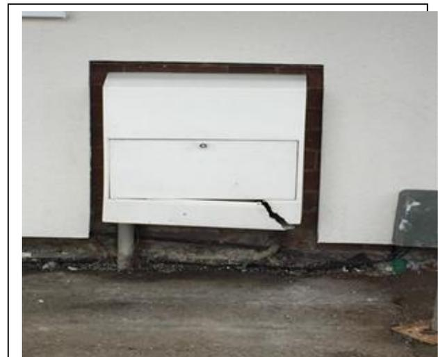
Fig 2. Another example of discontinuous insulation which will result in temperature differentials in the structure and may result in condensation and mould growth problems.
