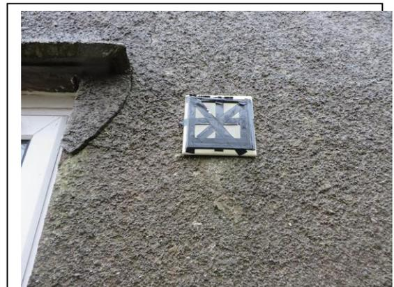
Fig 6. An example of an intermittent fan which had been covered by the occupant. In many instances the alterations may not be so obvious.
