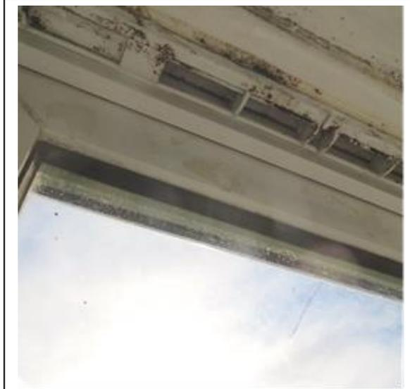
Fig 7. The picture above shows a trickle vent which was stuck to the window frame but without sufficient opening.
